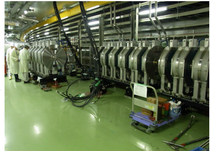
Photo of ①~③ cavities installation in 2015
