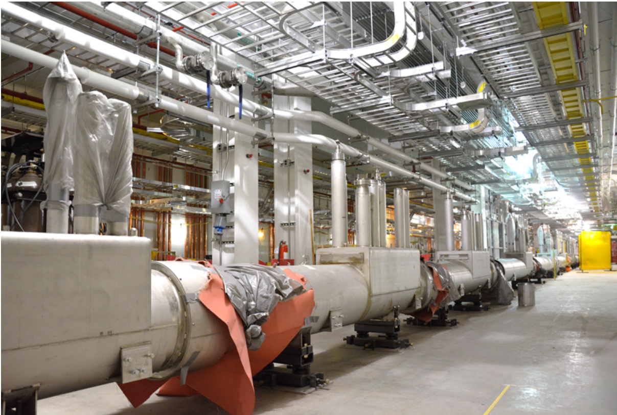
Transfer line installation in Linac Tunnel
