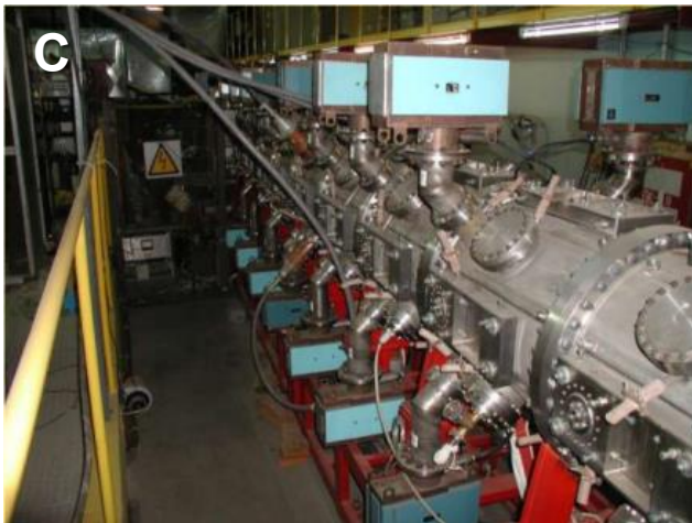
Heavy Ion Injector, 81 MHz, A/Q=3 (ITEP, Moscow)
