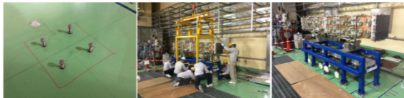
Holes drilling and anchoring installation
