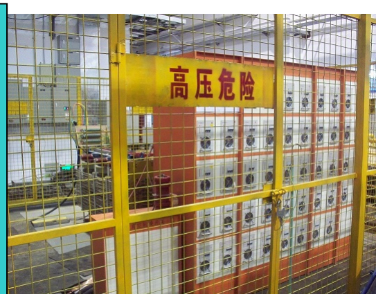
PSM 48 modules in serial configuration
